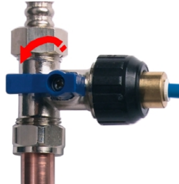
4) Turn on the water to the filter
